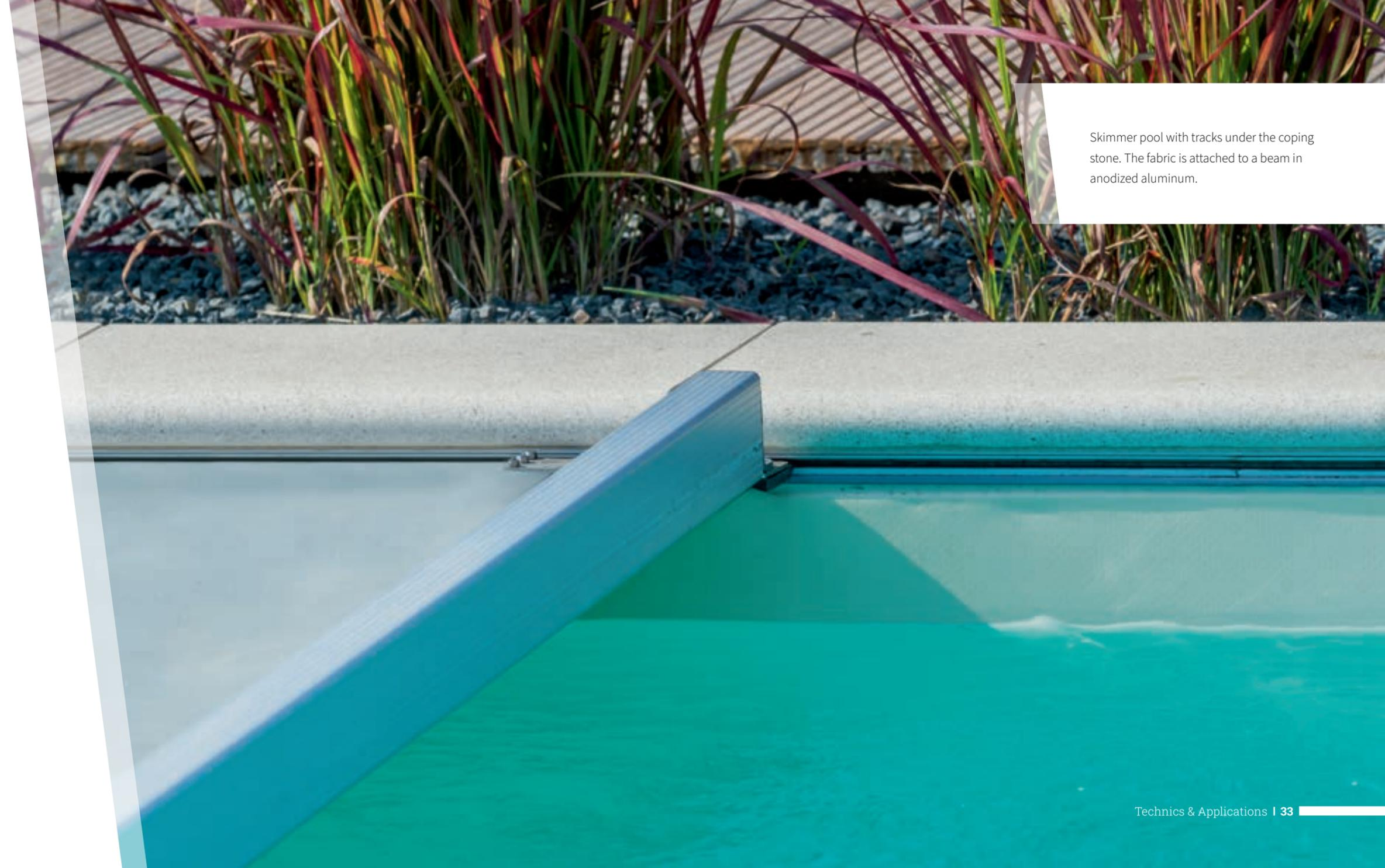
Skimmer pool with tracks under the coping stone. The fabric is attached to a beam in anodized aluminum.
